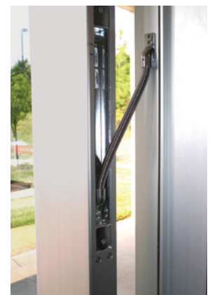
EPT (Electric Power Transfer) mounted to door in retrofit application
